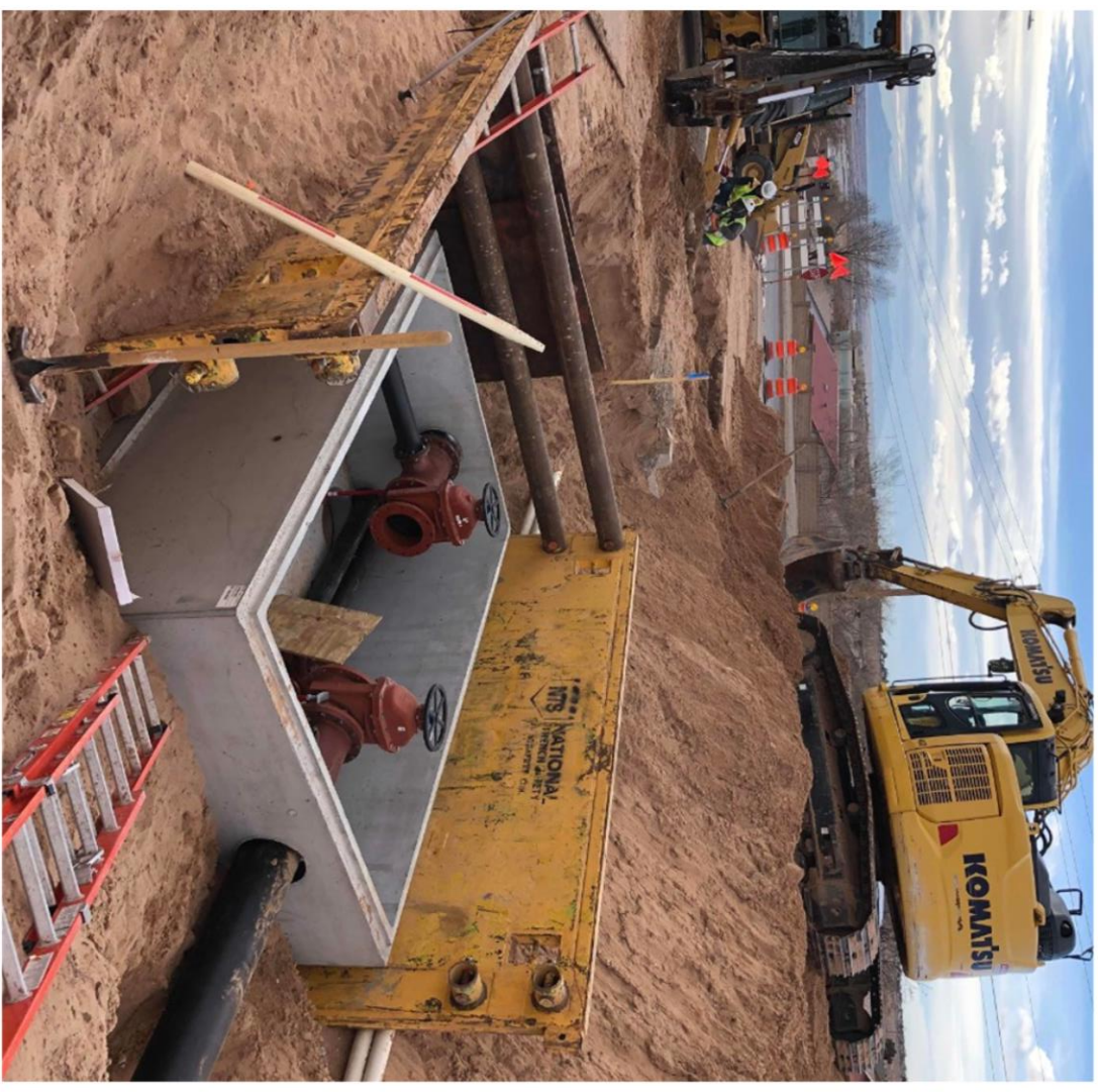
City of Rio Rancho Road Project
